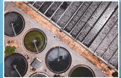
Water Treatment Reverse Osmosis Solvent Extraction
