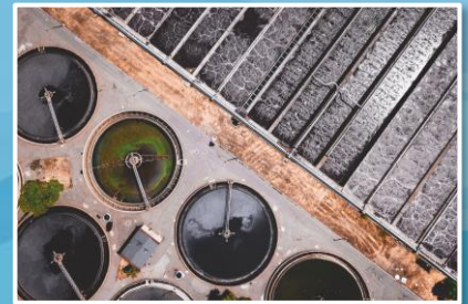
Water Treatment Solvent Extraction Reverse Osmosis
